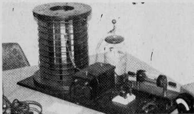
An early spark telegraph transmitter also entered in the old equipment contest at AWA Conference. The Rolling-pin shaped glass tube holds the spark gap apparatus.
