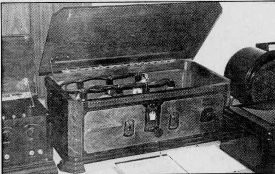
This Metrodyne receiver is one of the first AC operated radios with the filament connections at the top ends of the tubes. In this photo you can see the filament harness running across the tops of the tubes. The lack of batteries was a boon to radio sales.
