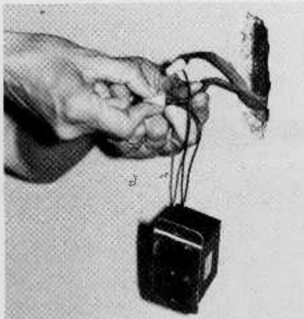
After cutting off power at the fuse box, remove the light switch and install Vigilite in its place. The whole job takes five minutes.
