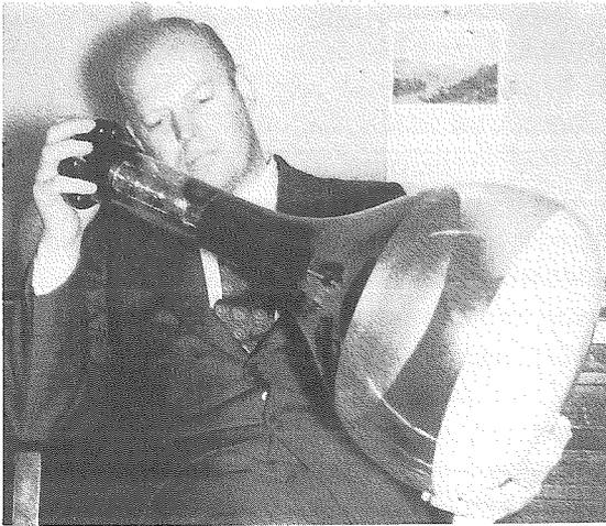
Figure 2.18 Dr. Du Mont holding 14-inch diameter electrostatic deflection cathode-ray tube as used in early television receivers circa 1939. (Courtesy of Jacob Ruiter.)
