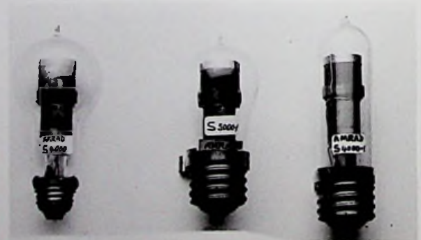
Amrad—the first gaseous rectifiers c. 1922.
