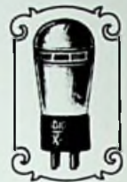
Radiotron UX-171
