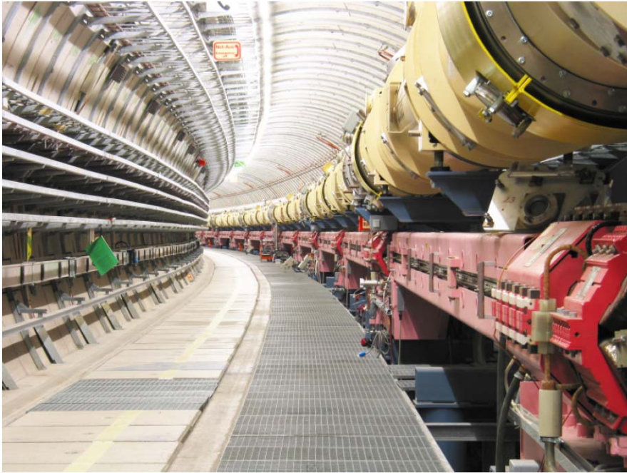
Fig. 8.1. View of the HERA accelerators, an electron/proton collider facility with a circumference of 6300 m and a bending radius of 800 m. The superconducting magnets for the 920 GeV proton beam are installed on top of the normal conducting magnets for the 27.5 GeV electron beam
