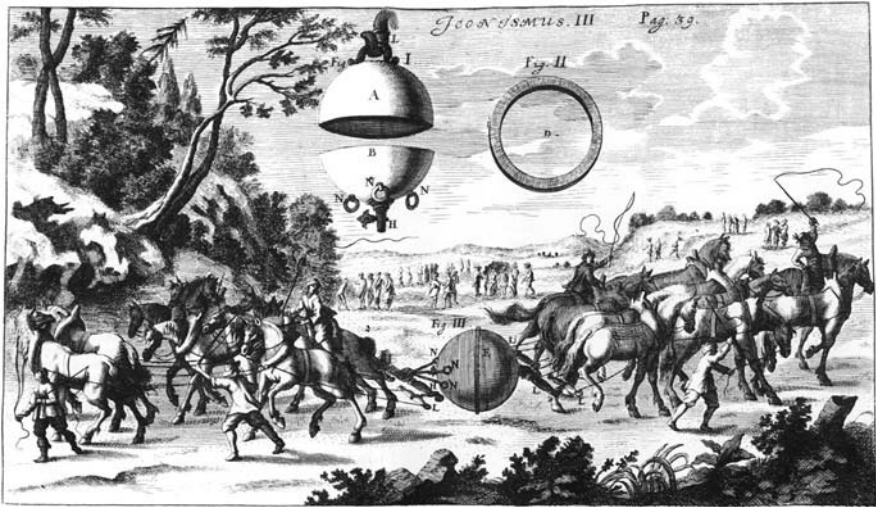
Fig. 11.1. Historical vacuum experiment of Otto-von-Guericke with the Magdeburg half-spheres [1]
