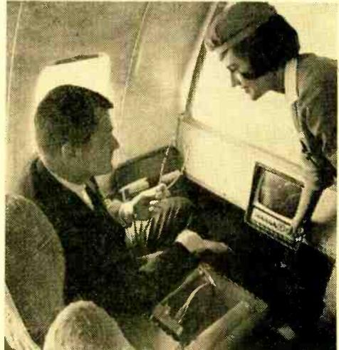
A stewardess instructs a passenger aboard an American Airlines Astrojet in the use of Astrovision, an in-flight entertainment system. At passenger's right elbow is earphone jack and sound control knob.
