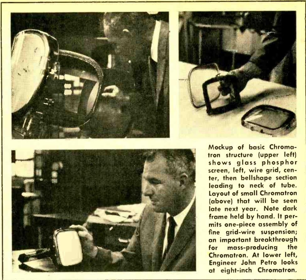
Mockup of basic Chromatron structure (upper left) shows glass phosphor screen, left, wire grid, center, then bellshape section leading to neck of tube. Layout of small Chromatron (above) that will be seen late next year. Note dark frame held by hand. It permits one-piece assembly of fine grid-wire suspension; an important breakthrough for mass-producing the Chromatron. At lower left, Engineer John Petro looks at eight-inch Chromatron.
