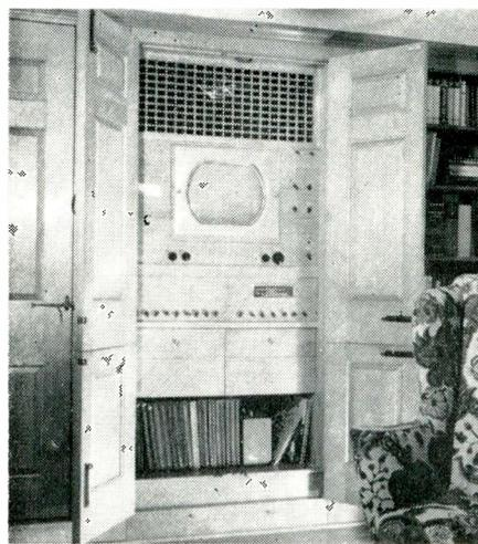
A top-notch custom installation featuring AM-FM tuner, hi-fi audio equipment, television, record players, and even an antenna rotator control.
