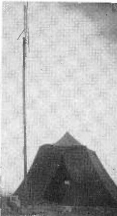
Equipment used by W6NJJ, holder of second highest score in the Test. The transmitter includes an HY-75 triode and Vibrapack Power Supply, Field-strength meter is also shown.
