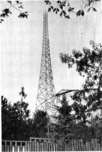
W6QBU's tower, complete except for rotary beam mechanism. Note ladder on right side.
