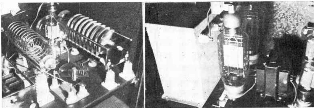
*Here is the Kalifornia Kilowatt at W6SZ in all its grandeur. It's an Eimac 450TL, operating as cold as a cucumber with 999.99 watts input. The modulator (right-hand illustration) likewise employs large tubes, but with conservative output, which is one of the reasons why W6SZ's speech quality is tops.*
