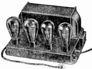
The PAM 85 is similar to the power amplifier stage of the PAM 80 and is designed to be operated from the voltage amplifier stage of the PAM 80. It has exactly the same power output and operating characteristics. Any number of PAM 85 power stages can be operated from the PAM 80, thus allowing the addition at any time of more power for any installation without discarding equipment previously purchased. Each PAM 85 comes with cord and plug to attach to the PAM 80 or to its preceding PAM 85.
