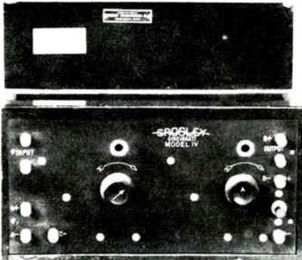
THE CROSLLEY MODEL IV (FOUR) WAS A 2-STAGE AMPLIFIER THAT SOLD FOR \$20 IN LATE 1923. IT WAS DESIGNED TO PAIR UP WITH CROSLLEY'S MODEL V (AND LATER MODEL 51) AND SHARED THE SAME CABINETS... AND WAS IDENTICAL TO ITS COUSIN, THE ACE 2-B.
