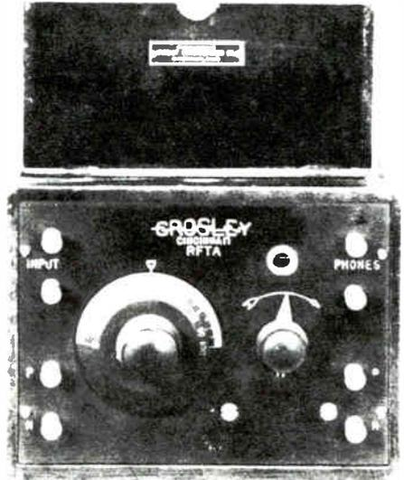
↑ THE RFTA UNIT WAS A RADIO FREQUENCY TUNED AMPLIFIER, WAS PRODUCED IN LATE 1922 IN THE NEWER-STYLED CABINET. ITS PURPOSE WAS TO ADD ONE STAGE OF RADIO FREQUENCY TO THE ALSO RE-STYLED HARKO.
